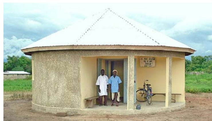
Newly built Health Station in a village in Côte d'Ivoire
