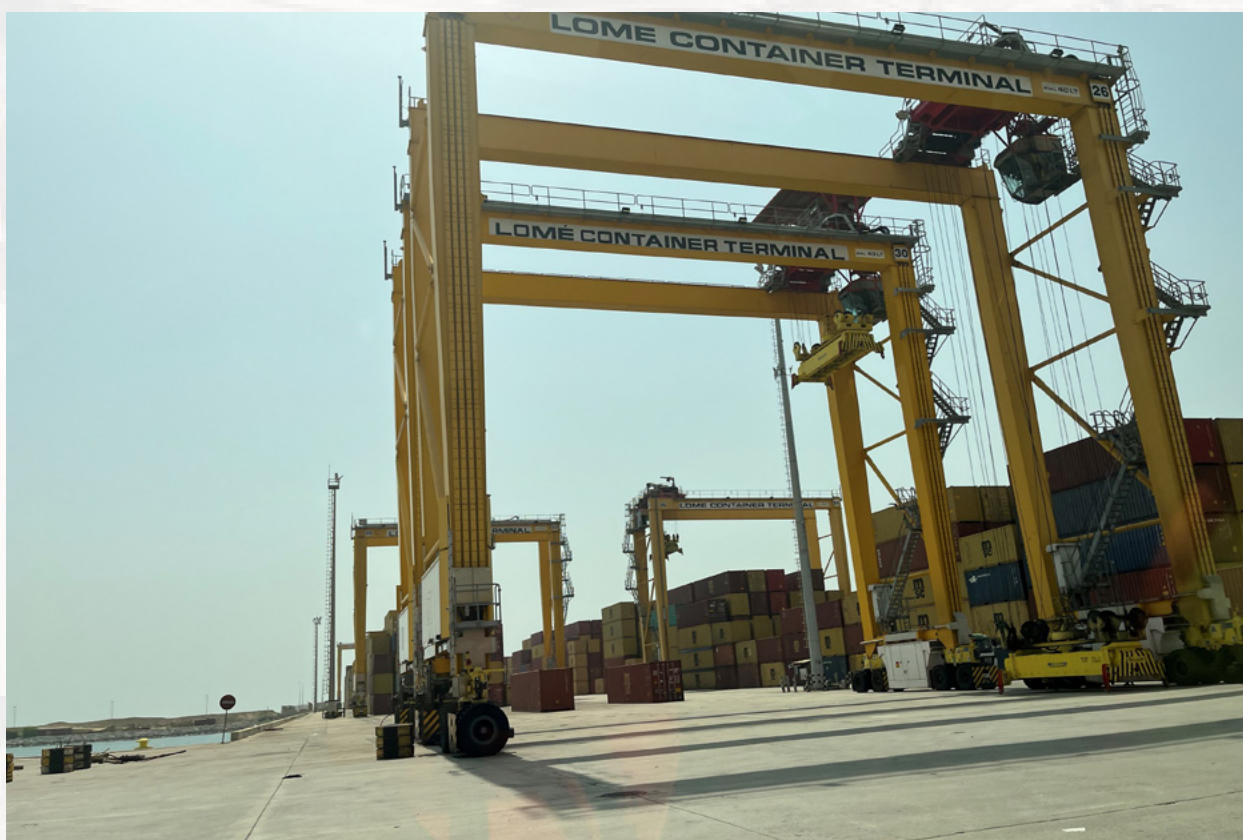
View from Lomé Container Terminal, December 2023.
