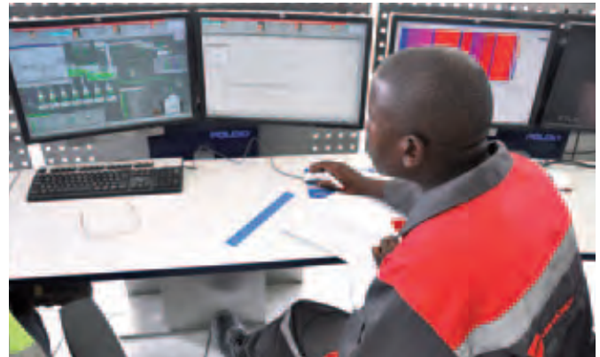
Control room of the cement production
