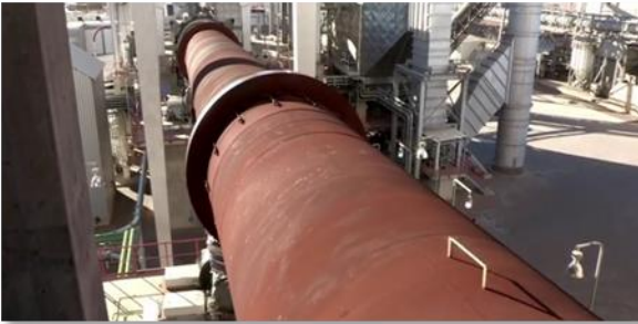
The rotary kiln at the Ohorongo plant
