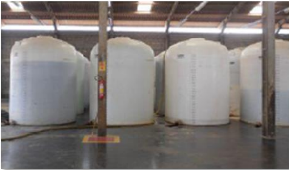
Storage tanks at ESDD: without containment wall
