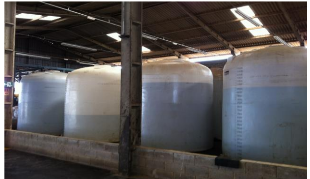
Storage tanks during visit: with containment wall
